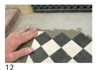
Continue around the perimeter of the chequer fitting all the triangles and using your level to check for straightness - also use your tape to measure the space/distance to the edge of the path from the newly created straight edge of the triangles and make sure the measurement remains roughly constant - a few mm difference is alright.
