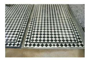
This type of anomaly in the pattern is also common with original Victorian floors. Sometimes the geometry works out and sometimes not. It's possible in certain cases to cut the sheeted border and stretch the design by spacing apart the mosaics a little or pushing them together slightly to make an exact fit around the perimeter with no overlaps in the pattern.
