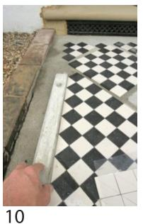
Scrape away the excess adhesive and lay your level alongside the triangles. Some of the triangles will need to be pushed in or out to meet the edge of the level to form a straight line. Look up and down the edge of the path top to bottom to check that a neat straight line has been formed.
